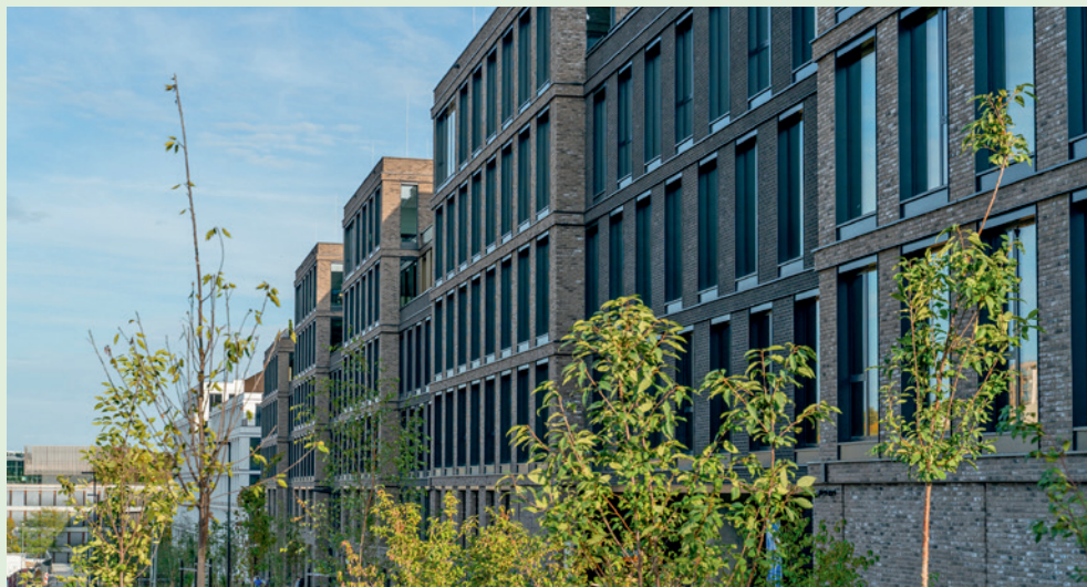
Nová Waltrovka – Legatica & Metalica, Prague 5 – Radlice ■ The project, finished in October 2023, was designed to meet the highest ESG parameters ■ Developer: Penta Real Estate ■ Technical Facility Management: Rilancio
