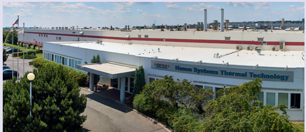
Panattoni Park Kladno South ■ Halls for Korean manufacturer Hanon Systems are already under construction Developer: Panattoni ■ Investor: Accolade
