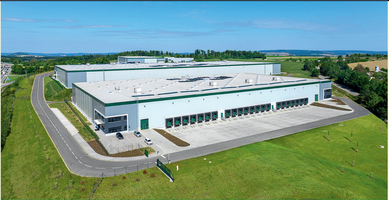
Prologis Park Ostředek (CR) ■ Developer: Prologis
