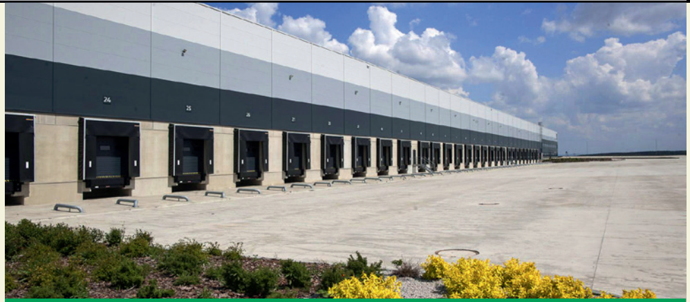
Prologis Park Pilsen II ■ Developer: Prologis
