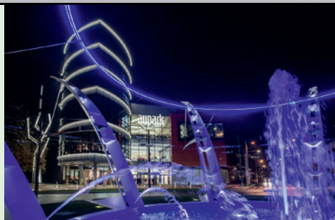
Aupark Hradec Králové Technical Facility Management: Rilancio
