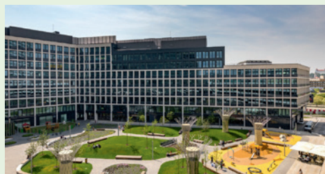
Pribinova 19 (part of Eurovea City) in Bratislava (Slovakia) was acquired by Prvý realitný fond managed by IAD Investments
